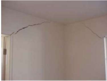
An example of large gaps in sheet rock
